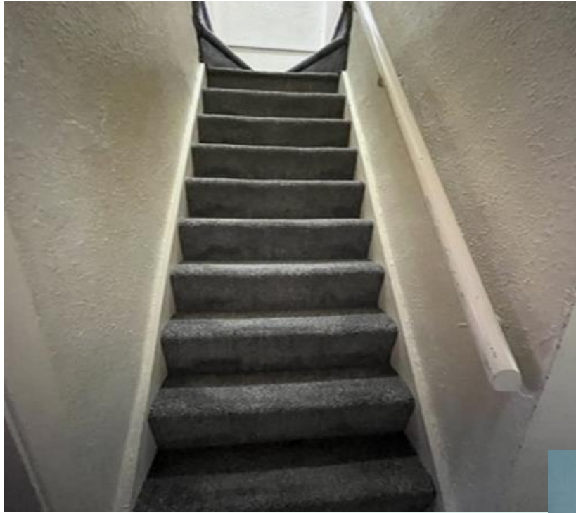
Category - falls on stairs
